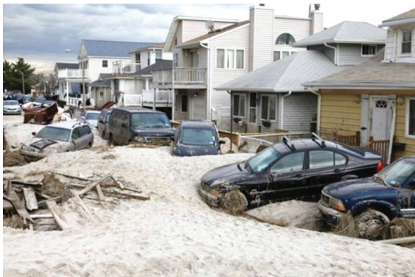
▲ Damage from Superstorm Sandy in Long Beach's West End, October 2012 (via NYRCR Long Beach Planning Committee)
